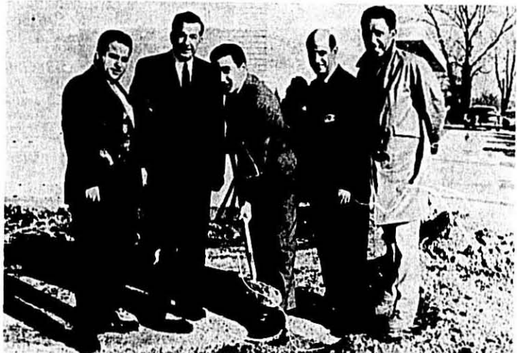
Prince Macaroni of Chicago, Inc., digs in to double the size of its Schiller Park, Ill., pasta plant. The new addition will add upward of 15,000 square feet to its manufacturing facilities besides increasing its warehouse area. Participating in ground-breaking ceremonies are (from left): Al Dubs, Prince sales supervisor; Weston Booth, Chicago manager of the Seavey & Flansheim Food Brokerage Co.; Anthony Costello, general manager of Prince; Frank Motta, Prince plant manager, and Joseph DeBartola of the Pilgrim Construction Co. Prince Macaroni of Chicago is a division of Prince Macaroni Mfg. Co., Lowell, Mass.
