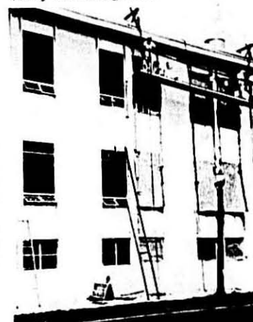
Workmen in process of applying second coat of white epoxy compound. Windows are carefully masked to protect them during application of paint.
