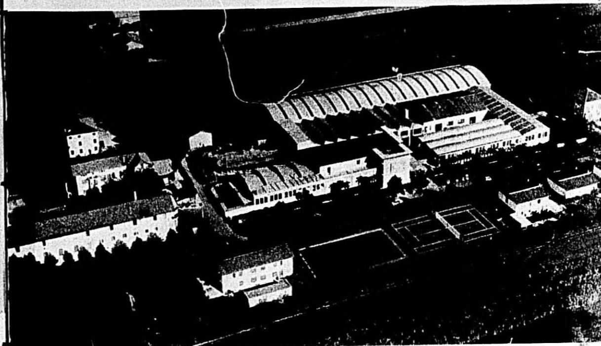
Air view of Pavan works
